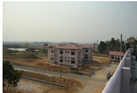
A View of Grade – IV Quarter
